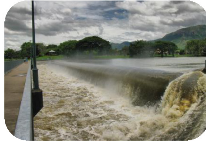
Flooding during an extreme storm in Sacramento
